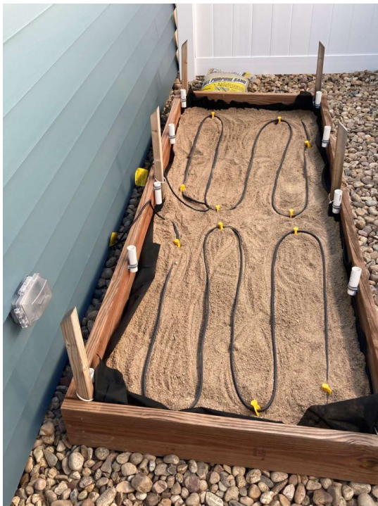
Figure 7 Cables set with tent stakes.
