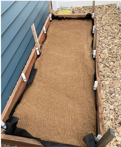
Fig 5. First Layer of Sand
